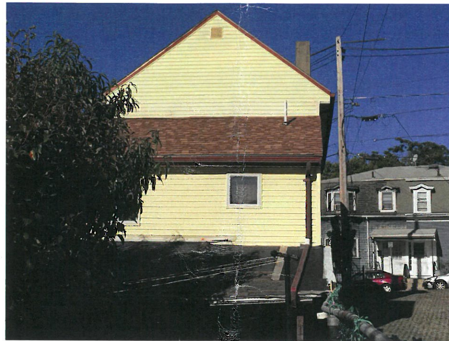
VIEW OF REAR
