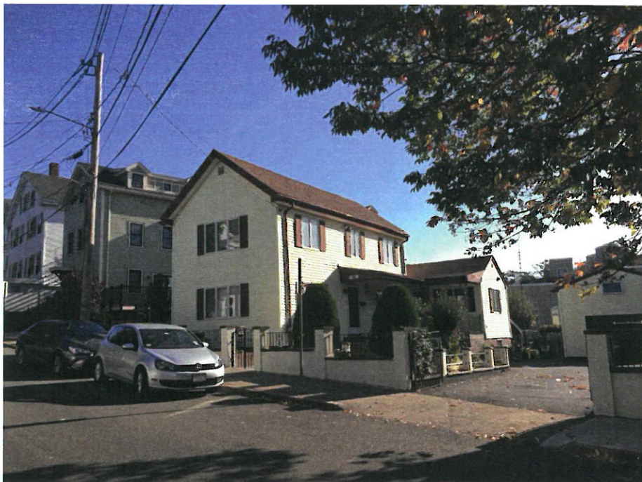
VIEW OF EXISTING HOUSE FRONT VIEW FROM RIGHT
